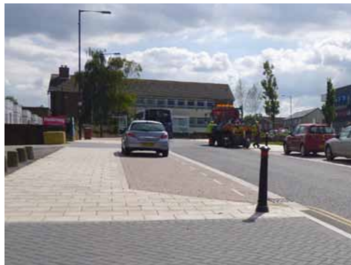
Concrete paving with red blocks in parking bays
