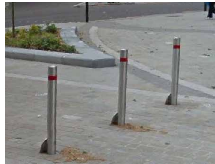
Stainless steel bollards with visibility bands
