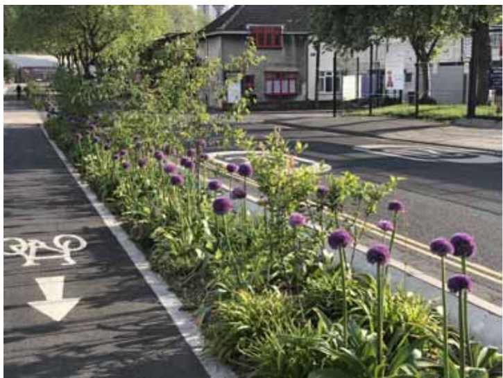
Raingarden with SuDS planting in Bristol
