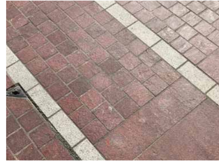
Red granite for benches with silver for kerbs
